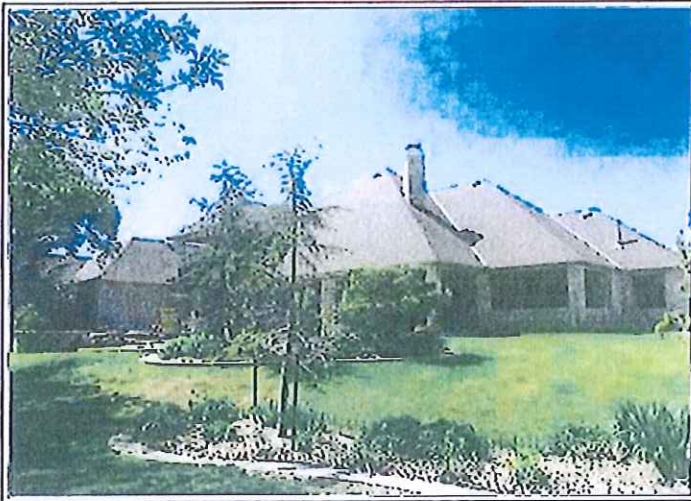
REAR OF SUBJECT PROPERTY
