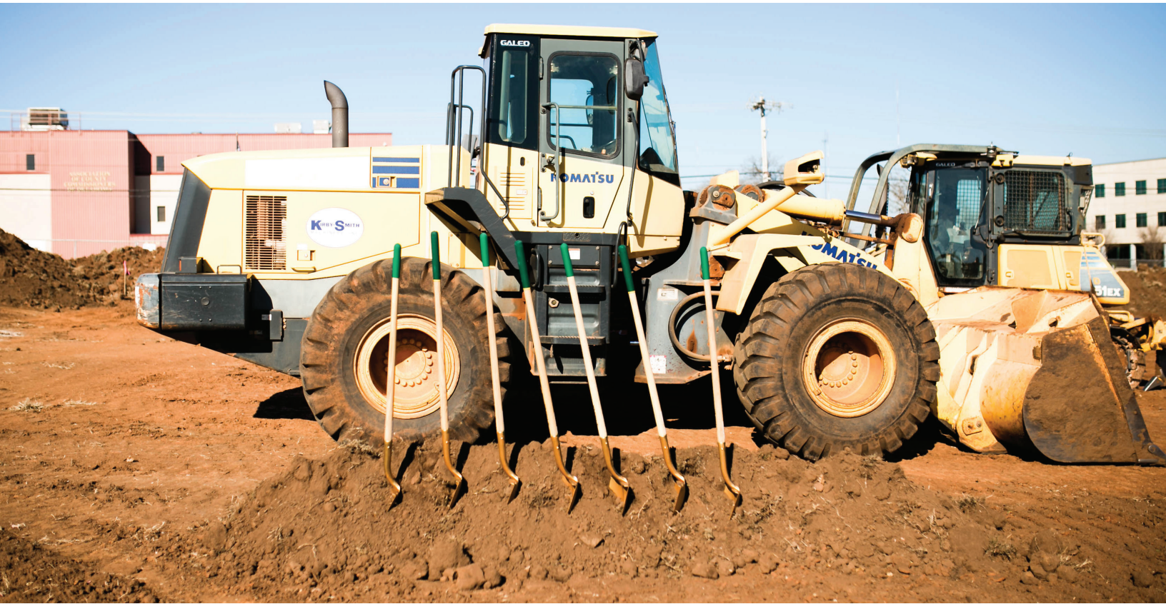
Ground breaking November 2018
