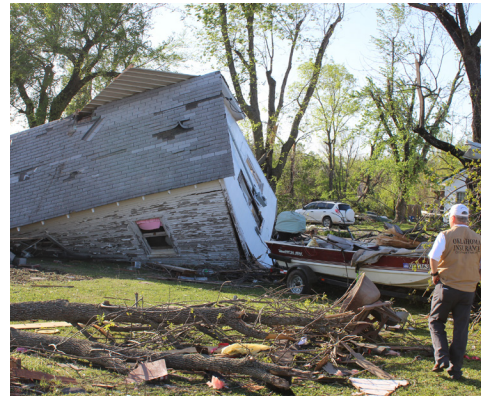
Commissioner Doak tours tornado damage in Quapaw.
