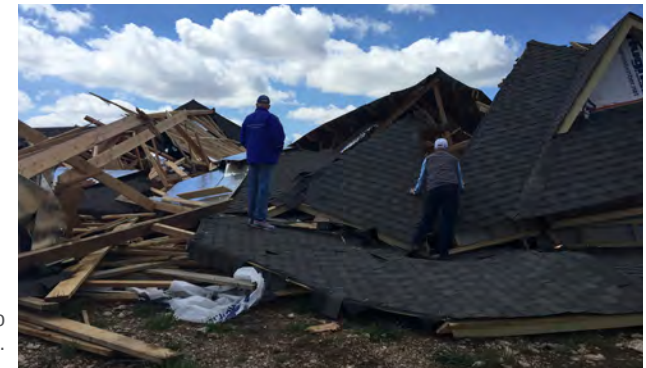
Commissioner Doak surveys tornado damage in Tulsa.
